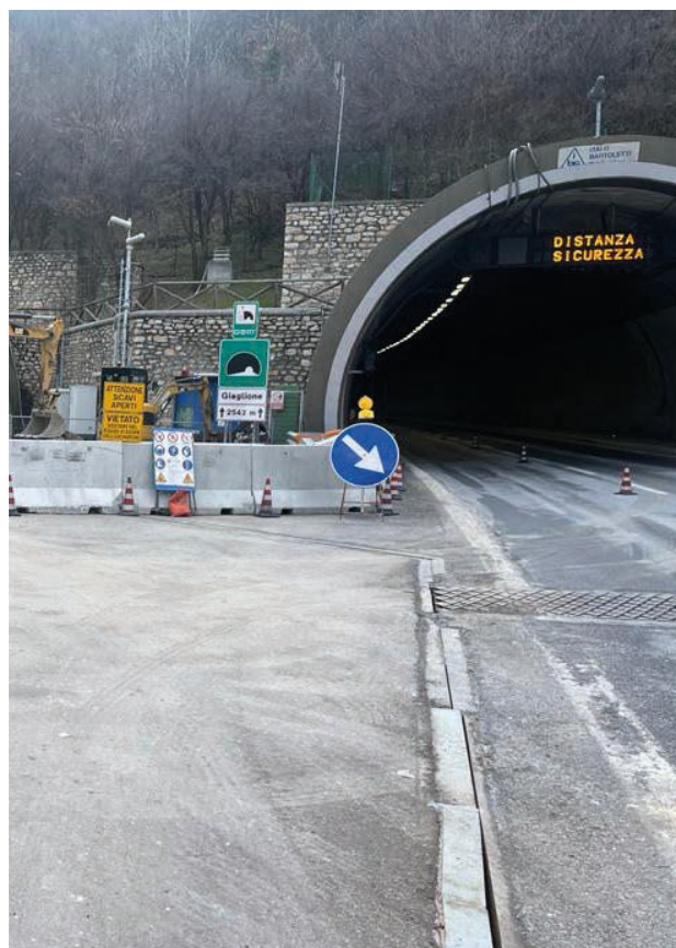
S.I.T.A.F. S.P.A - Giaglione and Ramat Tunnels
