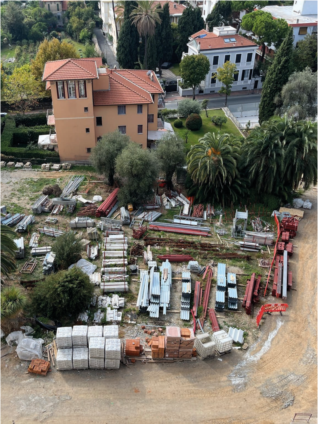
GSKD EDILE S.P.A -ANGST - Renovation Technological Systems Housing Complex , Bordighera
