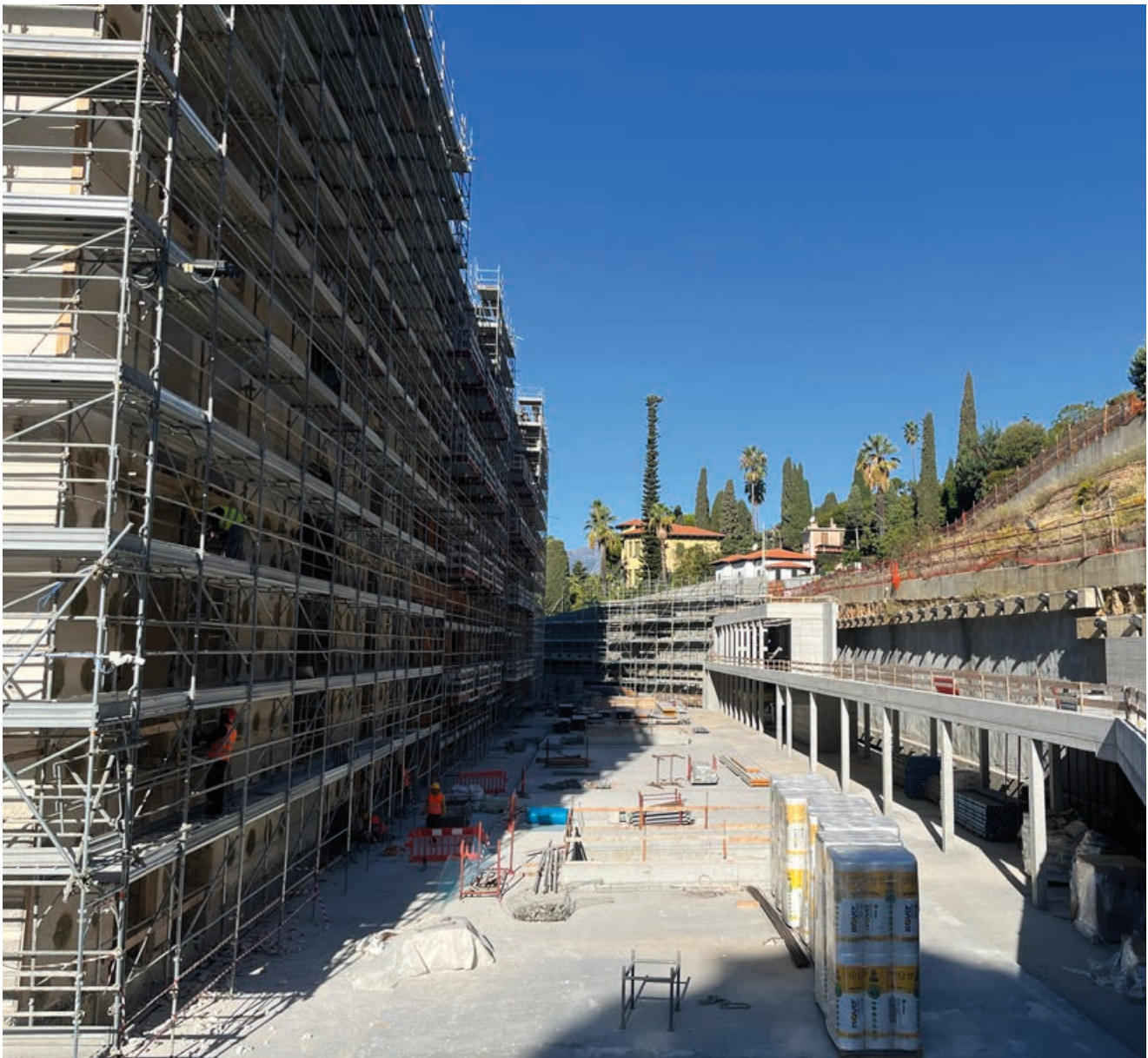
GSKD EDILE S.P.A - ANGST - Renovation Technological Systems Housing Complex , Bordighera
