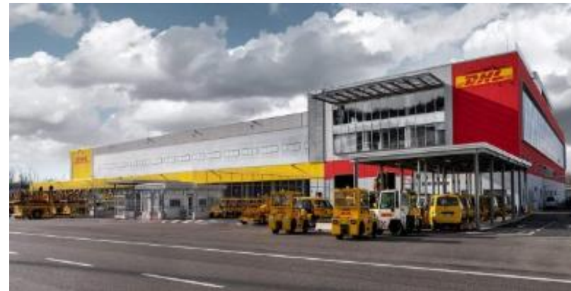
Client: DHL EXPRESS (ITALY) S.R.L. Description: Electrical and special electrical systems for the realization Hub DHL Express- Malpensa.
