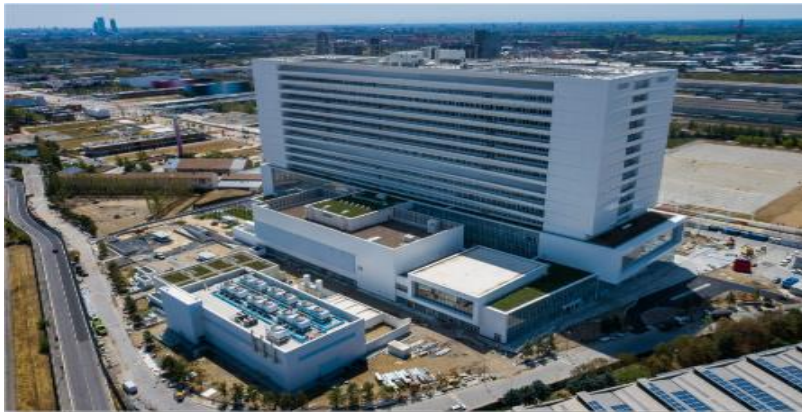
Client: GKSD EDILE S.P.A. Description: Engineering services and implementation of electrical and mechanical plant for the new Galeazzi Hospital, Milan
