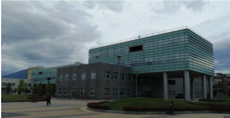
Client: UNIVERSITY OF NAPLES Description: Upgrading of University of Napoli
