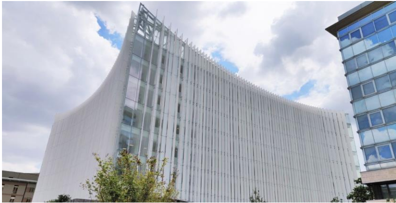
Client: OSPEDALE SAN RAFFAELE S.R.L. Description: The New Surgery and Emergency Hub of San Raffaele Hospital, Milan
