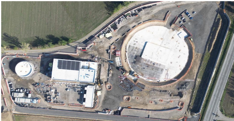
Client: CODELFA S.P.A. Description: Execution of electrical and mechanical systems of the new sports hall in Tortona
