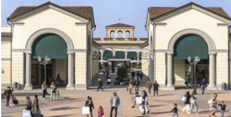
Client: SERRAVALLE VILLAGE S.C.A.R.L. Description: Construction of electrical and mechanical systems for the construction of the multipurpose and commercial building
