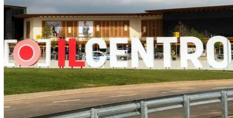
Client: TEA S.p.A. Description: Implementation of electrical and mechanical systems for the Arese shopping center
