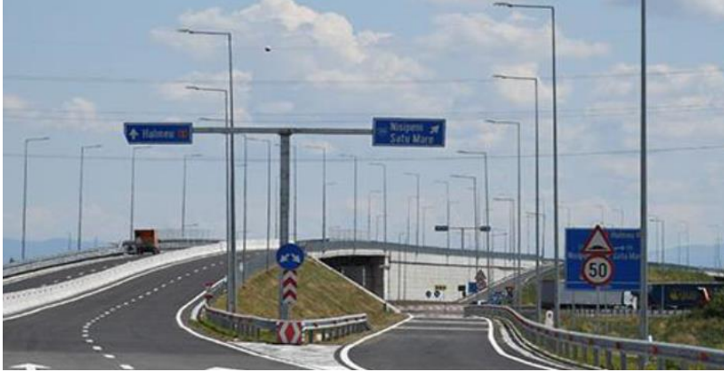
Client: COMPANIA NATIONALA DE ADMINISTRARE A INFRASTRUCTURII RUTIERE S.A. Description: Lighting Installations Satu Mare Bypass, Romania
