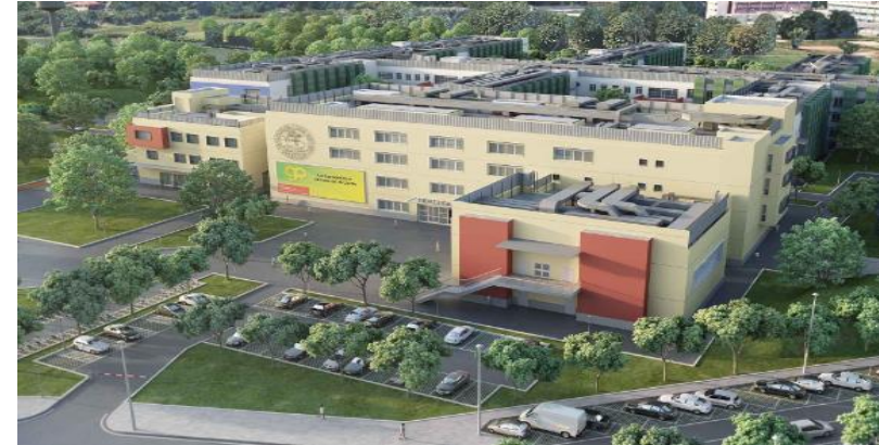
Client: UNIVERSITY OF TURIN Description: Design, financing and implementation of the New University Area of Grugliasco
