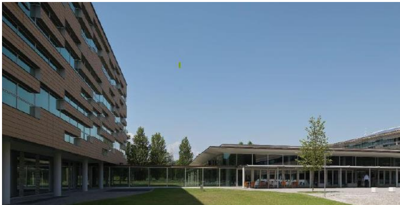
Client: CASSA DI RISPARMIO DI PARMA E PIACENZA S.P.A. Description: Supply and installation of electrical and Mechanical systems for Cariparma Business Center.
